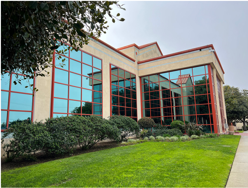
The view from the driveway of the administration building at the Chevron El Segundo Refinery.
