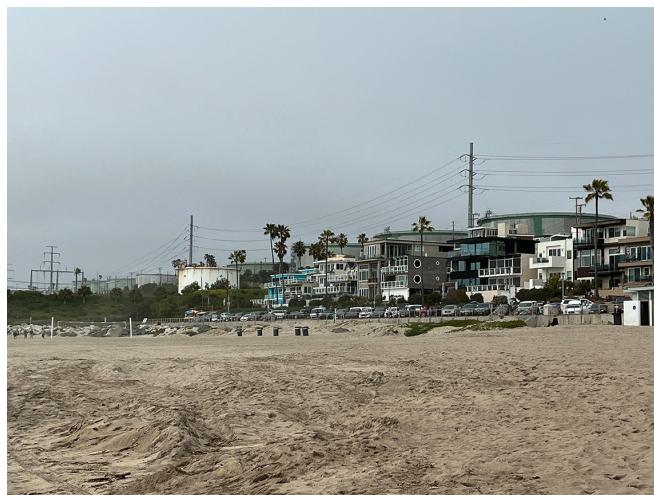
The view from Manhattan Beach of green-painted refinery tanks behind beach houses.
