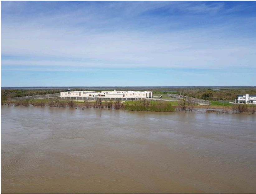
The Plaquemines Parish Detention Center was rebuilt on the same Louisiana marsh for $105 million after Hurricane Katrina destroyed the original building. Map data © March 2019 Google. Image uploaded by nomad.
