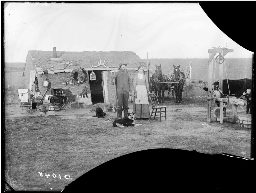
“‘Nebraska Gothic,’ the John Curry sod house near West Union, Nebraska,” 1886. Courtesy of Nebraska State Historical Society [NBHIPS 10236].
